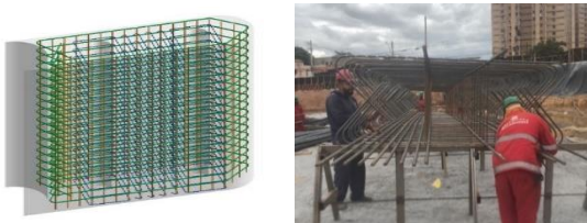
Figure 9. Modeling the reinforcements' panels and assembling them on-site.
