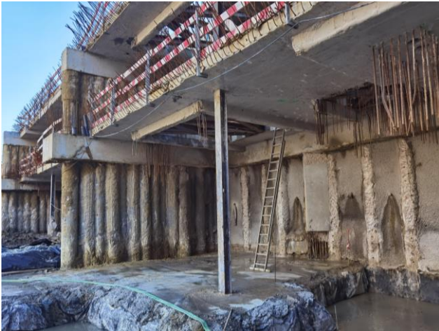
Figure 6. Concrete slab strips supported by HEB200 micropiles and buttresses.
