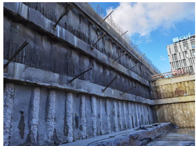
Figure 5. Bored pile wall shored by temporary ground anchors.
