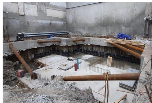
Figure 4. The spacer system of the pit at the stage of excavation to the bottom of the pit.
