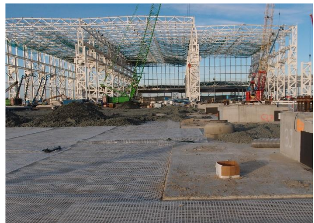
Figure 7. 1st installation level of the geogrid reinforcement.
