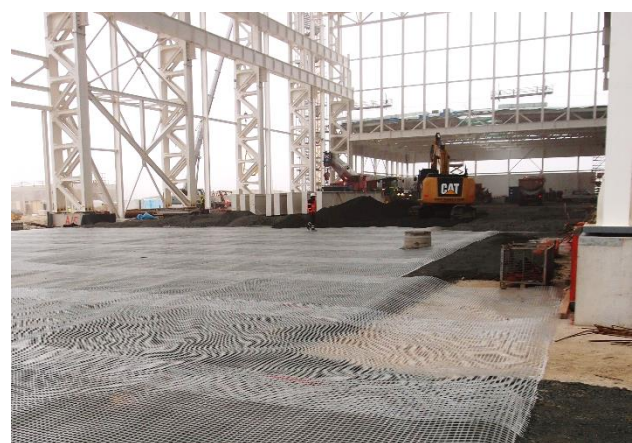
Figure 8. 2nd installation level of the geogrid reinforcement in the production hall area.
