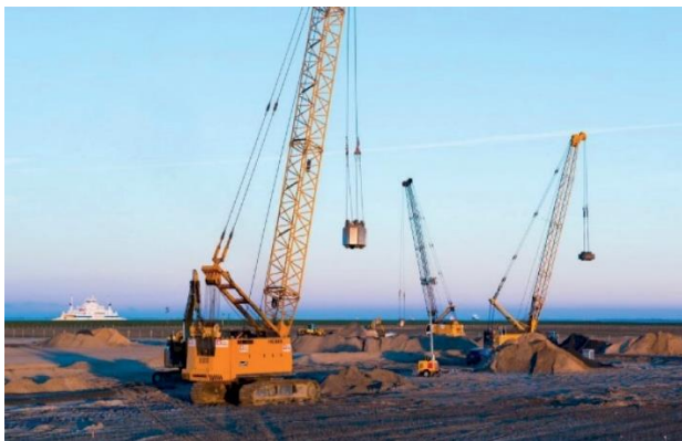
Figure 3. Execution of dynamic compaction.
