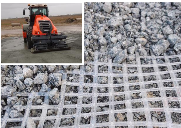
Figure 6. Interlocking of base course material and geogrid, compaction with the help of plate compactors (2 nd installation level).
