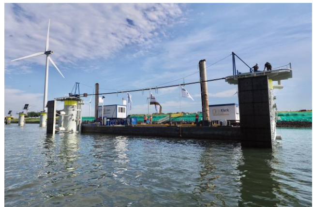
Figure 1. Test setup, pile 81-D04 (left) and 81-D01 (right).
