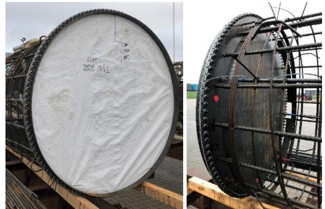
Figure 2. Flat-jack system used for the E3006 project.
