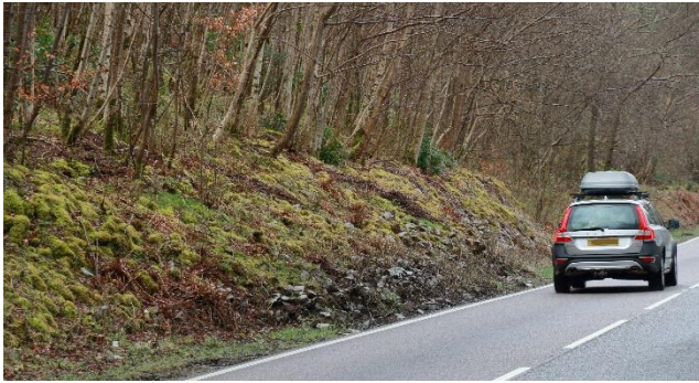
Figure 4. The original distance of the toe of the bund from the edge line of the carriageway was approximately 2m, by April 2022 the distance had reduced to zero in places.
