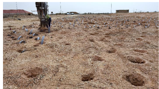
Figure 3. Installation of the prefabricated vertical drains.
