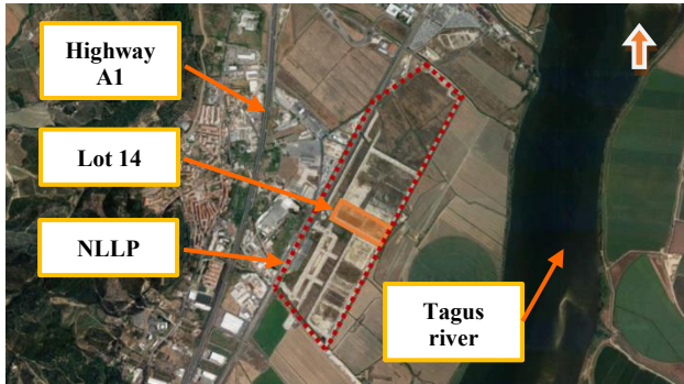
Figure 1. Aerial view of the construction site (image taken from Google Earth).
