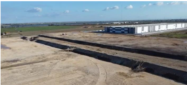
Figure 5. Aerial photograph of the pre-load embankments.
