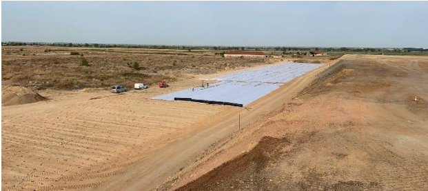
Figure 4. Aerial photograph of the drainage geocomposite installation.
