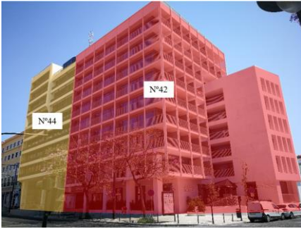
Figure 1. Reinforced concrete buildings above de tunnel.
