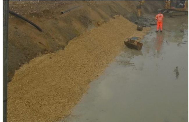
Figure 9. Construction of angular stone key.
