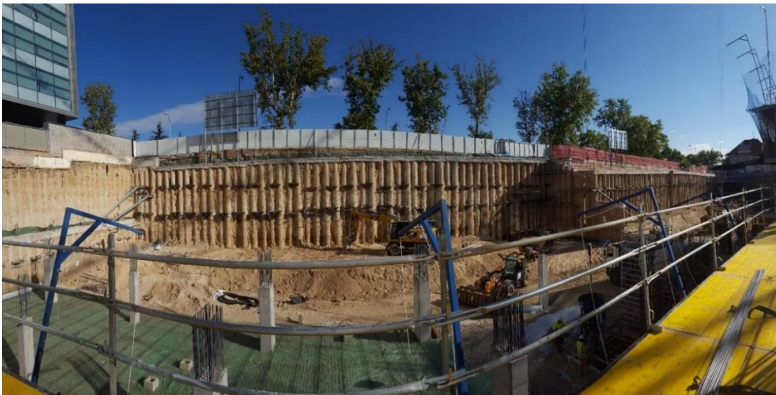
Figure 1. Front view of the retaining wall during the construction works (©Arup).
