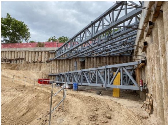
Figure 2. Front view of the strutting system (©Arup).
