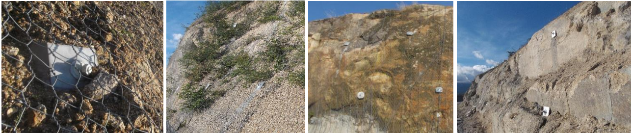
Figure 2. Examples of slope stabilisation in granitic rock masses that have different weathering levels and joint patterns.
