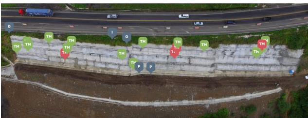
Figure 4. Critical asset network of sensors using icons (TM-tiltmeters, I-Inclinometers, P-Piezometers, O-Other) and colours (Green-sensors are OK, Red-alarm threshold and Gray-no connection).
