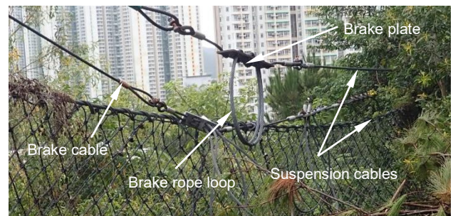
Figure 2. Longitudinal cables and brake elements.
