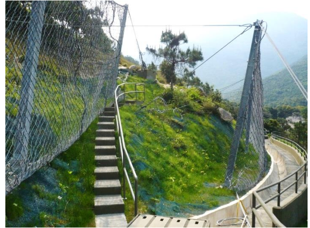
Figure 1. General view of barriers FW-1A (left) and FW-1B (right) after installation in 2012.
