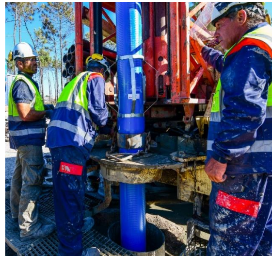
Figure 9. Drilling of deep dewatering borehole.
