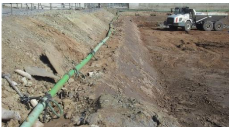
Figure 2. A site with appropriate groundwater control.
