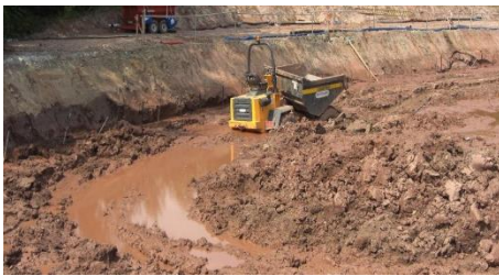
Figure 1. A site without any groundwater control.
