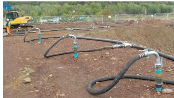
Figure 10. Series of pressurised recharge boreholes.
