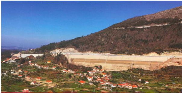
Figure 1. General view of the M24 embankment, reinforced with soil-cement.
