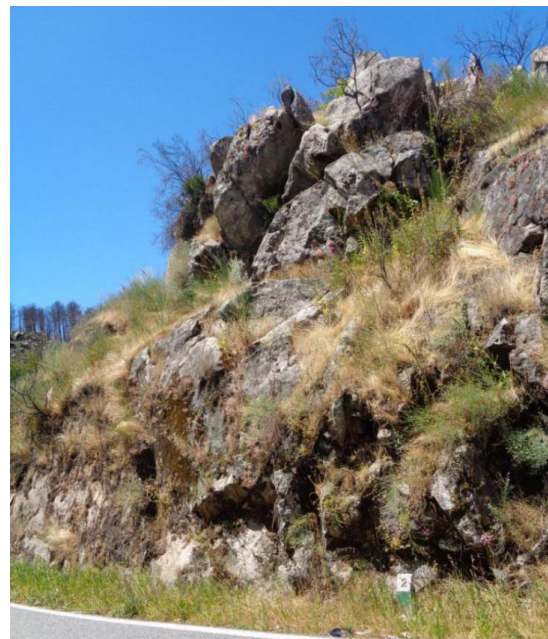
Figure 2. Slope featuring loose blocks with kinematic potential.
