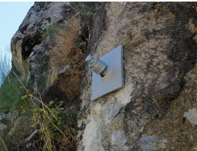
Figure 9. Application of punctual nailing in excavation slopes.
