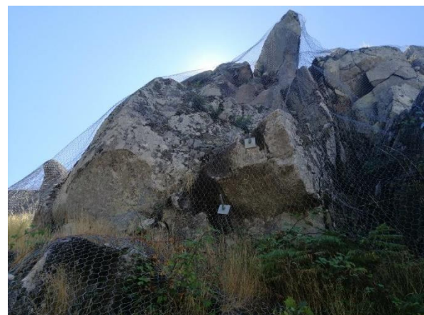
Figure 7. Application of triple twist net and nailing in excavation slope.
