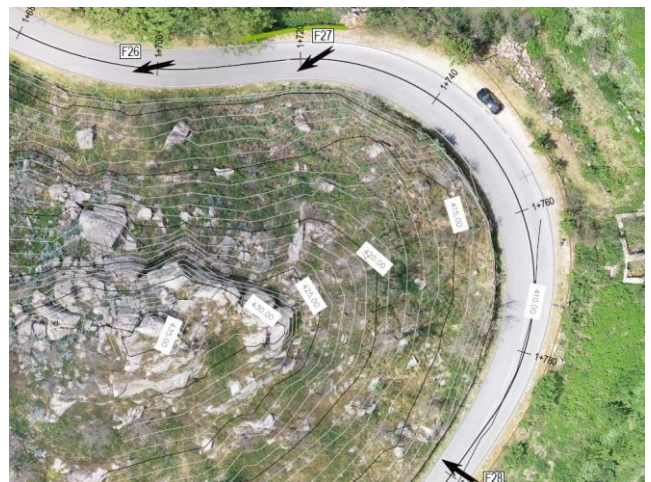
Figure 3. General aerial view of the site under study.
