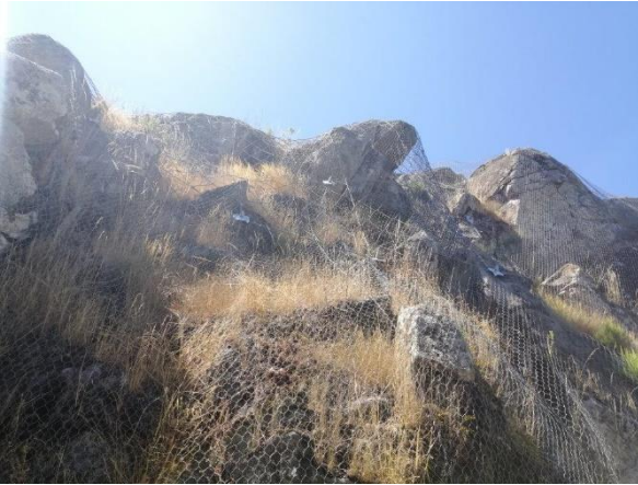
Figure 8. Application of HEA panels and nailing in excavation slopes.
