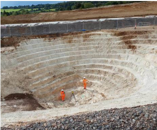
Figure 8. Excavation to base of feature at 'EM-S'.
