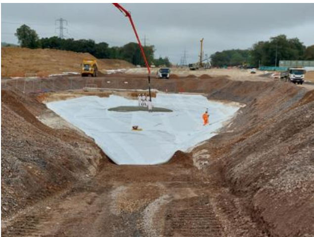
Figure 9. Installation of concrete plug at 'EM-S'.
