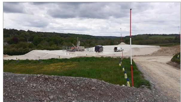
Figure 1. Completed trial embankment.
