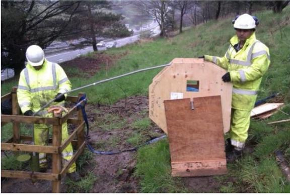
Figure 3. Automatic inclinometers (ShapeArray) installation.
