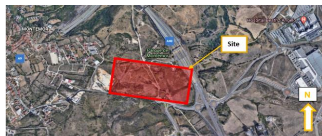
Figure 1. Site identification (Google Earth image).
