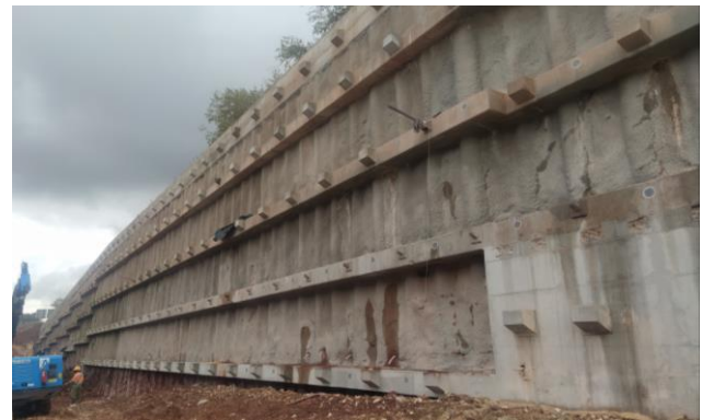
Figure 6. Excavation works near the bored pile wall.
