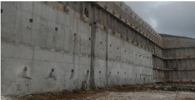
Figure 7. Excavation works near the concrete berlin-type retaining wall.
