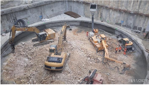
Figure 4. Transition between the square and circular section shafts.
