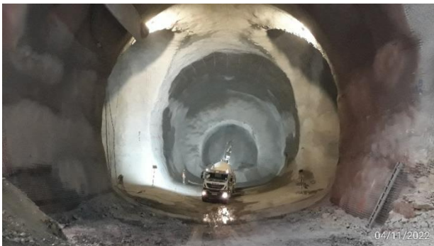
Figure 11. Southern station section showing in the middle the double track tunnel and side niches for the stairs and elevators.
