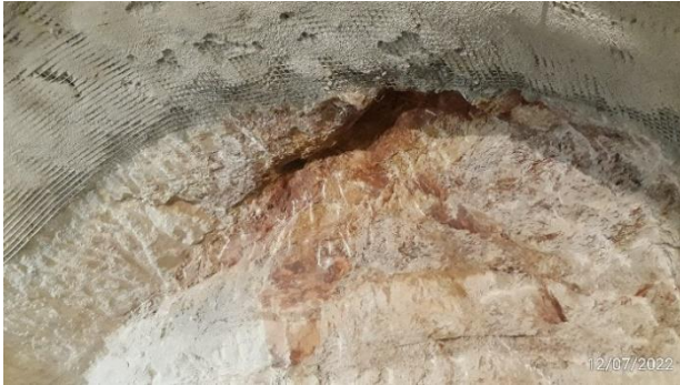
Figure 9. Fault materialized by the reddish-brown clay.
