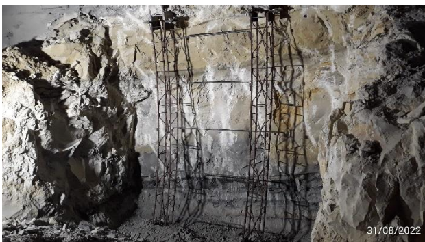
Figure 10. Lattice girders extensions at bench height, where the limestone-clay transition is clearly visible.
