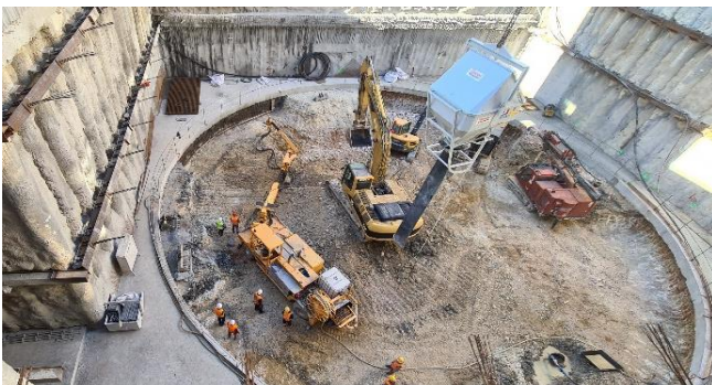
Figure 6. Piled retaining wall and the transition slab to the circular section shaft.
