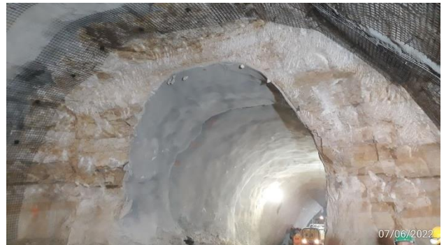
Figure 8. Pilot tunnel section against the station top heading section.
