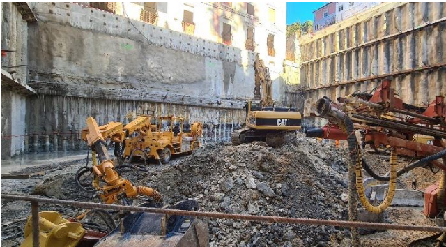
Figure 5. Upper piled wall with temporary ground anchors.
