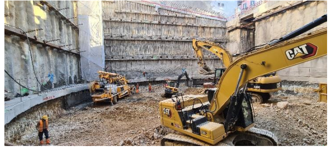
Figure 7. Micro pile retaining wall and beginning of excavation of circular section shaft.
