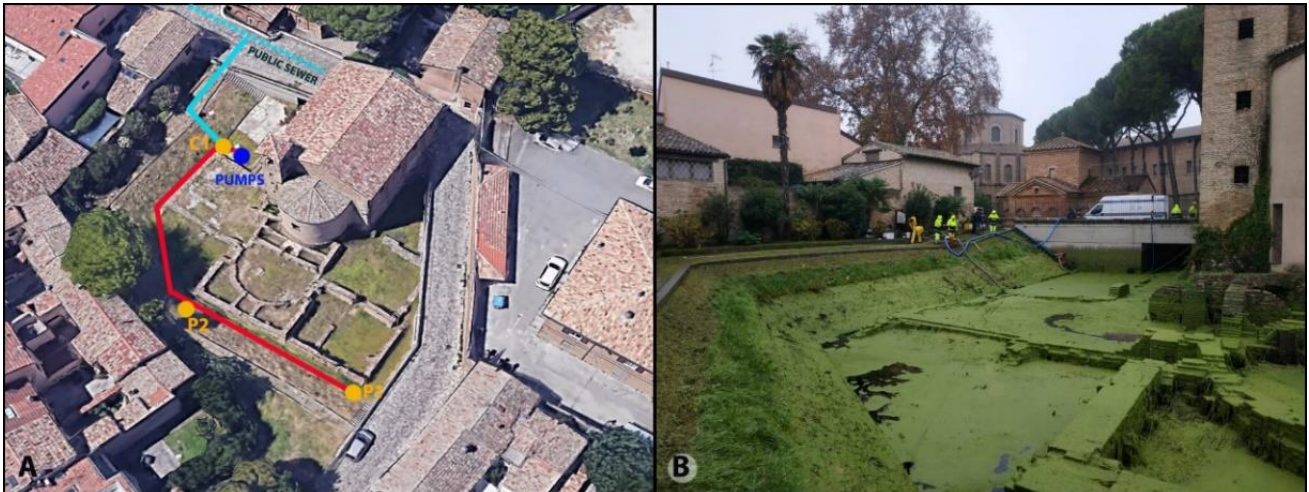
Figure 2. On the left, scheme of the drainage system operating in the area. On the right, a picture taken during the drying procedures required following the basin's flooding caused by the malfunction of the two submersible pumps in 2021.
