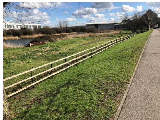
Figure 4. Current photos of the embankment showing high water table – water ponds in close vicinity of the embankment (on Thames River side).
