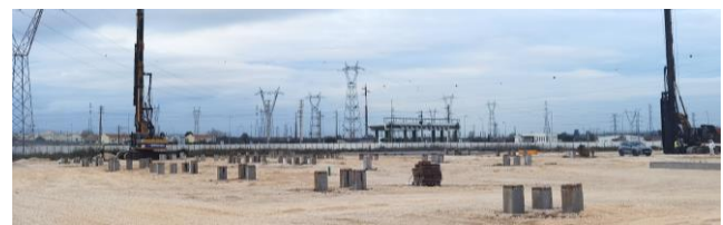
Figure 2. Driven piles.
