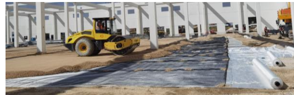
Figure 5. Load transfer platform.
