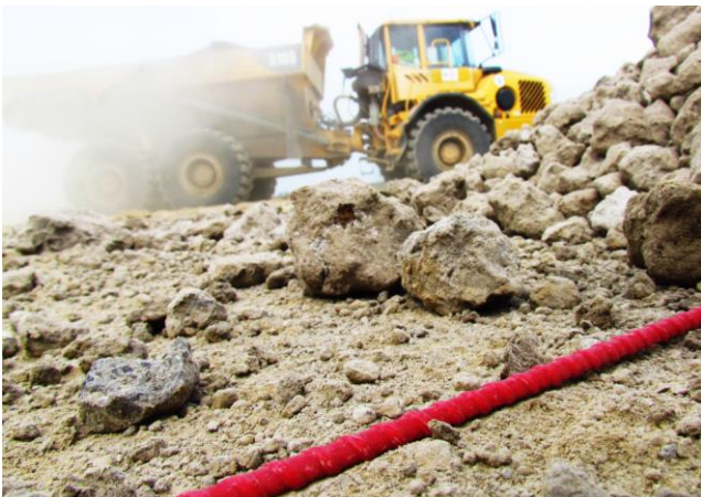
Figure 4. Challenging field conditions during embankment construction.
