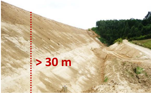
Figure 7. The view of the road embankment in question during construction.
