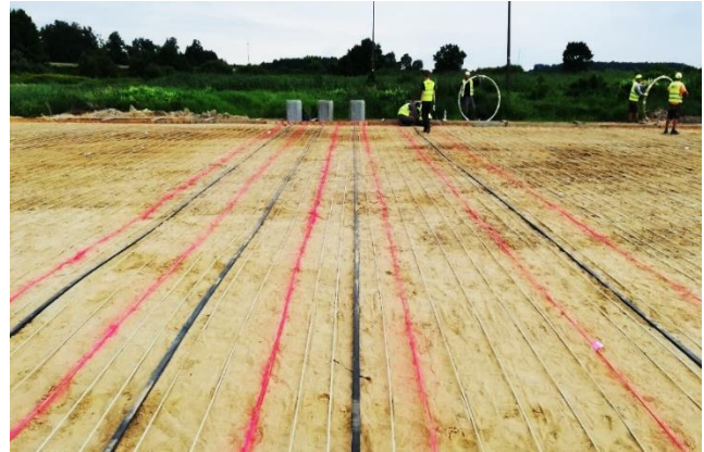
Figure 14. Installation of EpsilonRebars and 3DSensors at the base of the embankment.
