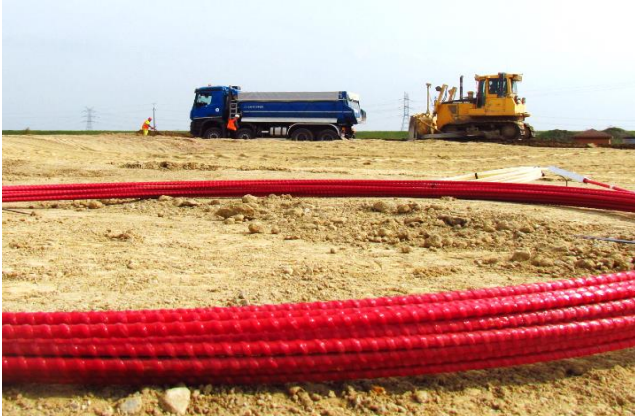
Figure 3. Monolithic sensor delivered on site in coil.
