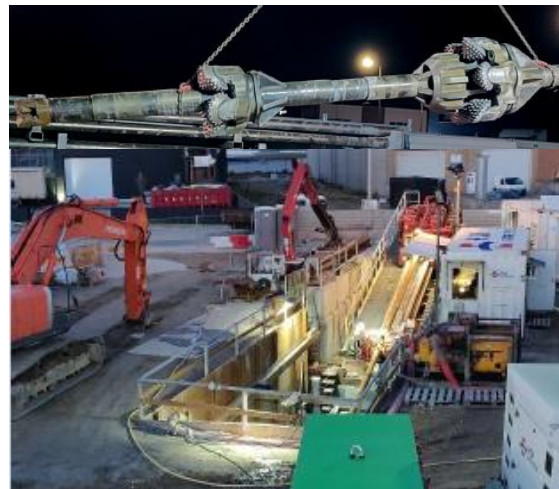
Figure 3. Forward reamer and launching pit.
