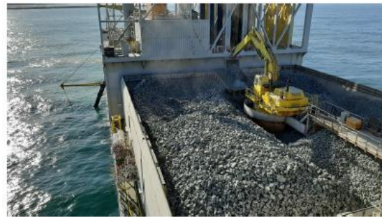
Figure 5. Rock berm construction operations (FPV).
