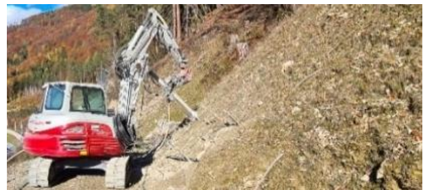
Figure 4. Installation of DCP-SBZ (self-boring tensile element) micropiles for testing purposes.
