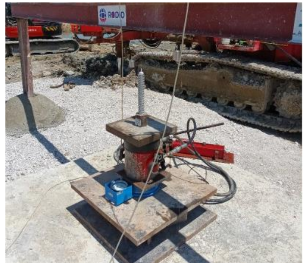
Figure 7. Full scale tension test: reaction structure view.
