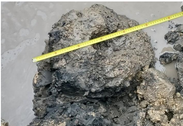
Figure 6. Trial column view.
