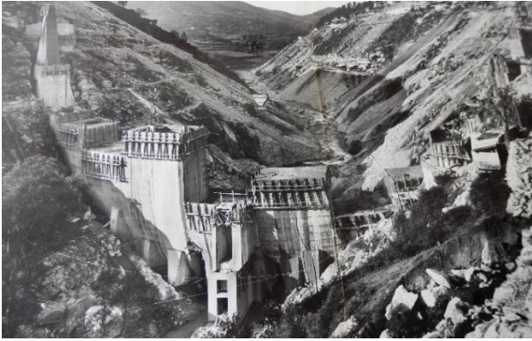
Figure 2. Construction of Caniçada dam reinforced concrete arch over granite bed rock (courtesy of Rodio).
