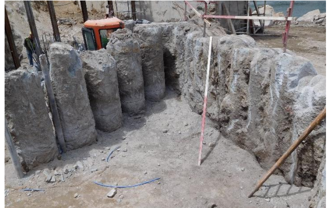
Figure 12. View of jet grouting excavated around columns.
