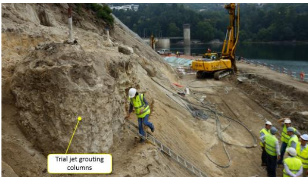
Figure 11. Trial column's view.
