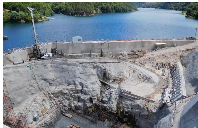
Figure 13. View of the excavation final works.
