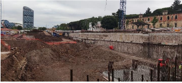
Figure 12. East Side solution with provisory anchors.
