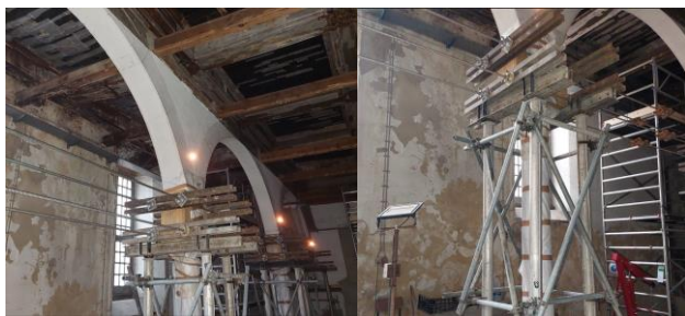
Figure 10. Internal bracing of the building's structure.
