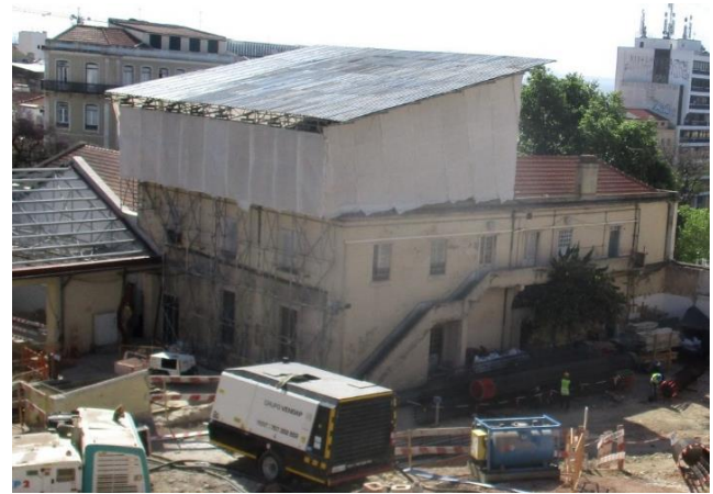
Figure 6. Low Choir (building’s exterior view).
