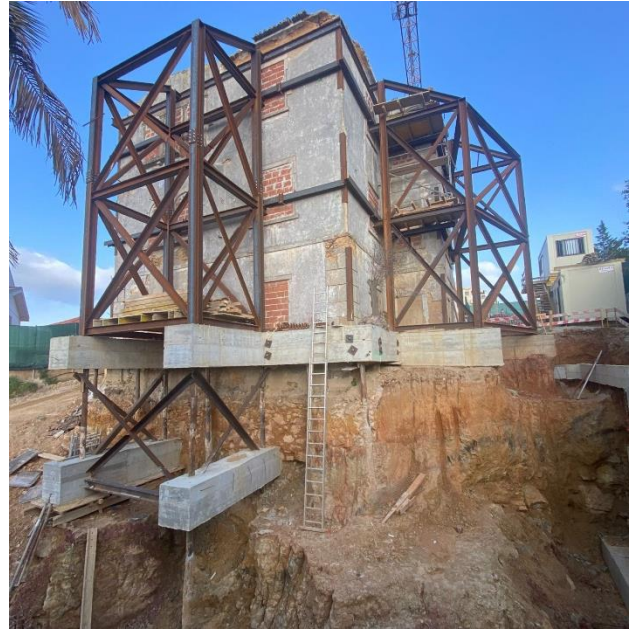
Figure 5. Facades retention and underpinning solution.
