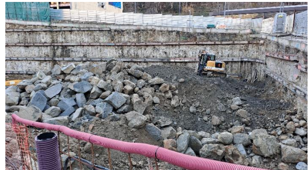
Figure 10. Some photographs of the retaining wall after the excavation of the site.
