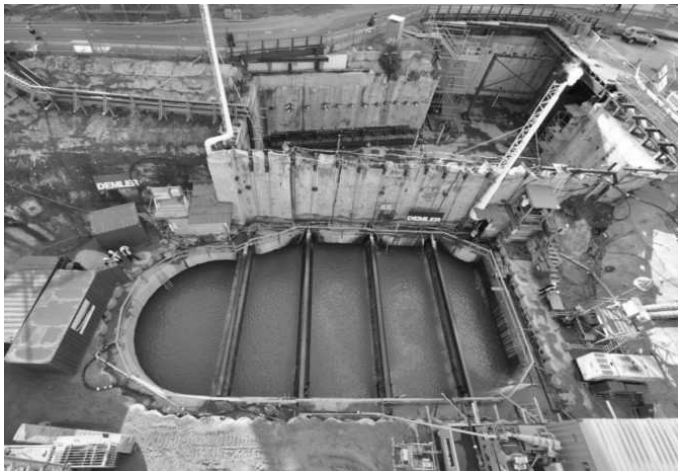
Figure 6. Salvage pit (in the foreground) in front of the eastern diaphragm wall of the 'GWB' pit.
