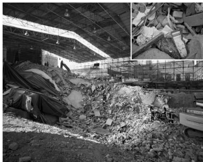
Figure 5. Salvaging the archives from the rubble of the collapsed Historical Archive at Waidmarkt, looking west with the eastern diaphragm wall of the 'GWB' pit.
