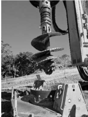
Figure 6. Spoil removal from casing
