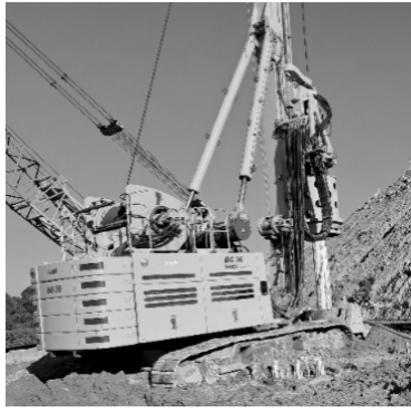
Figure 5. Bauer BG 36 Piling rig
