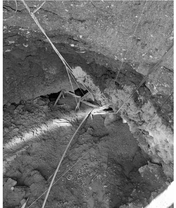
b) Grout bags after they have been pumped full of grout
