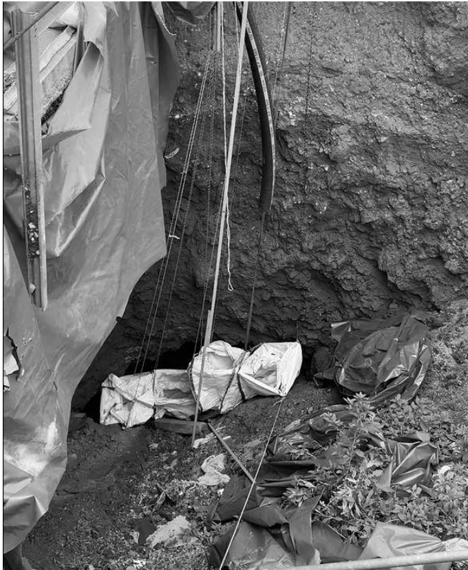
a) Initial placement of the grout bags in the throat of the sinkhole
