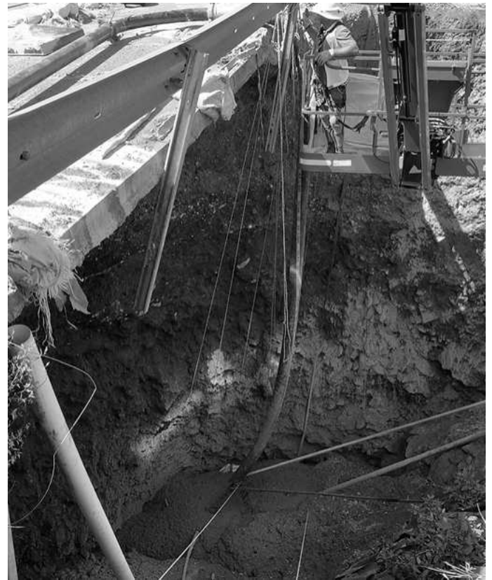
d) Pouring of the capping layer over the filled grout bags
