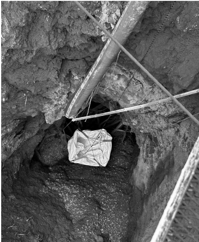
c) Placement of additional grout bags
