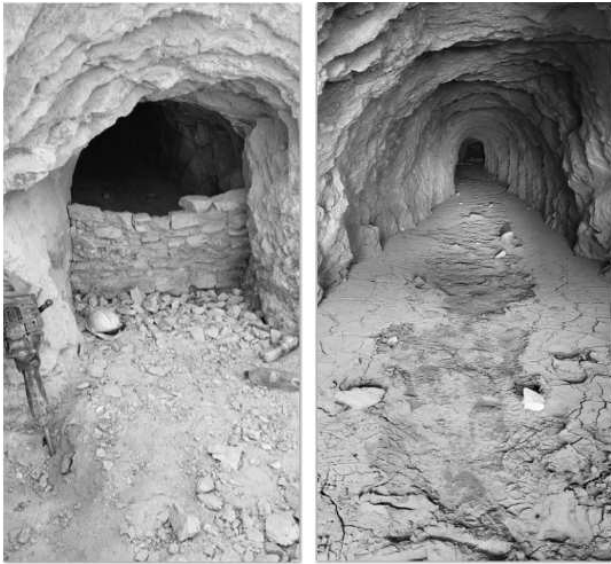
Figure 1. Exposure of an adit (access) tunnel approaching the mine stope from the north beneath Anderson Street
