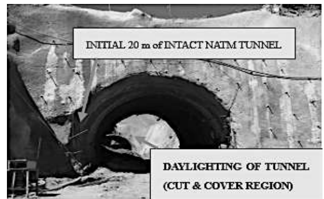
Figure 11. Complete Daylighting of Tunnel b/w Ch:1700 -1722
