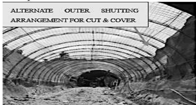
Figure 12. LG, Wire mesh & GI sheets for Gentries' outer shuttering Gantry
