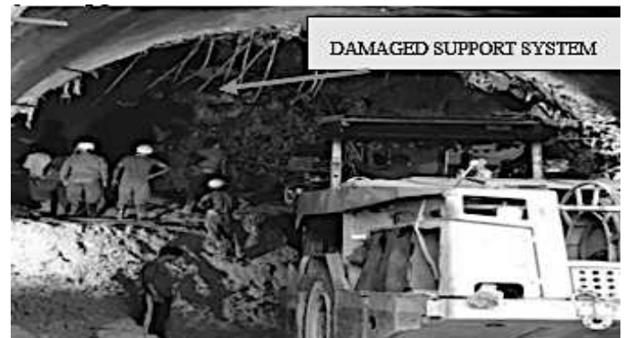
Figure 10. Damaged LG, Fore poles, Wire Meshes at RD 20m
