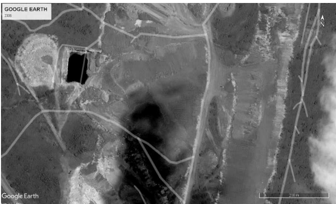
Figure 2. Case study – Open area showing the grey and brown surface materials (bordered by yellow dashes) of the pit and waste dumps – Google Earth image dated 2005
