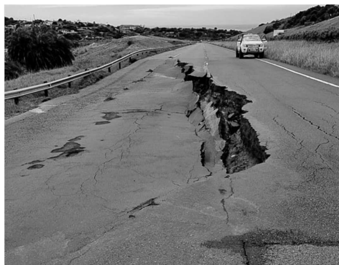
Figure 3. Slope failure at Site A
