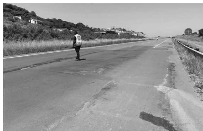
Figure 4. Site A before failure showing previous repair works due to movements
