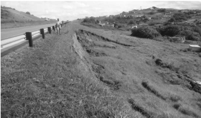
Figure 6. Slope failure at Site C
