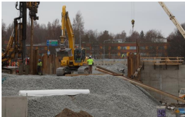
Figure 2. Up to 8 m high FGA embankment between sheet pile walls during bridge construction worksite at E12 highway (Auvinen et al. 2013).
