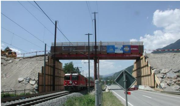
Figure 6, Temporary GRS in Switzerland using locally Fill Material and Soldier Beam Method
