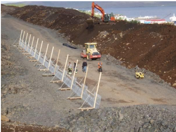
Figure 9 Installation of the first row of facing panels.
