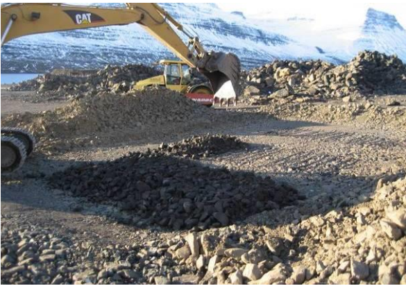
Figure 7 Installation damage trial.
