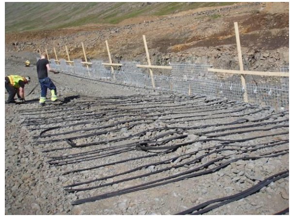
Figure 10 Laying out the soil reinforcement.
