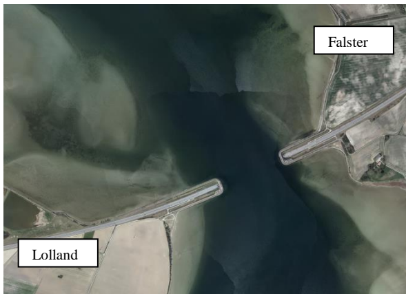
Figure 1.1. Guldborgsundtunnel. Aerial view.
