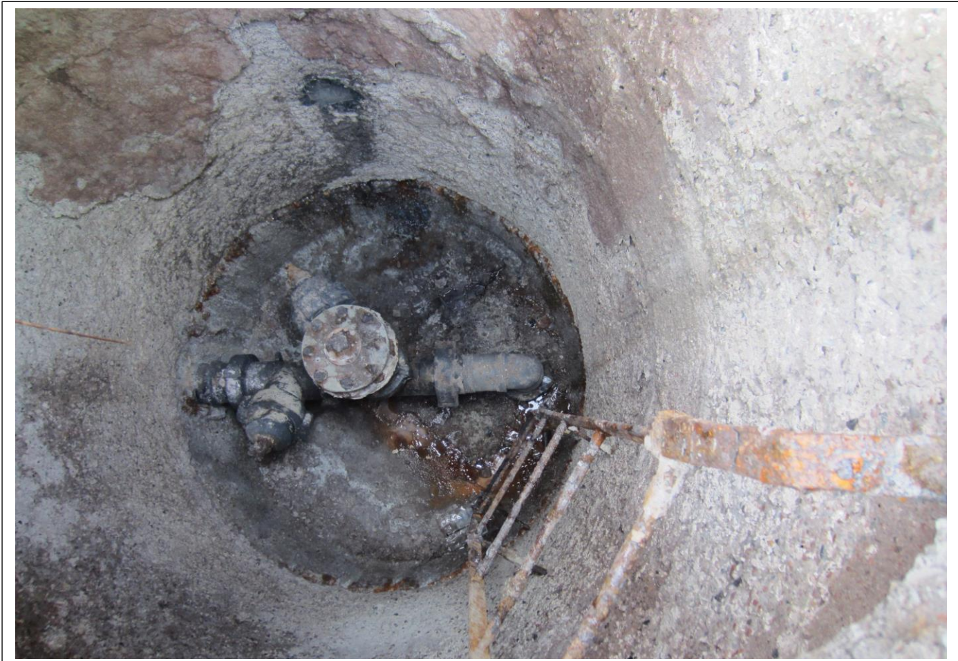
Figure 1.8 Installation of relief well in concrete ring on ramp at Lolland. Photo T.N. Petri.
