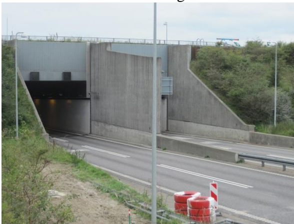
Figure 1.2 Photo from Falster site of tunnel entrance.
