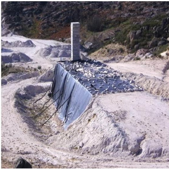
Figure 1 View of the experimental embankment.
