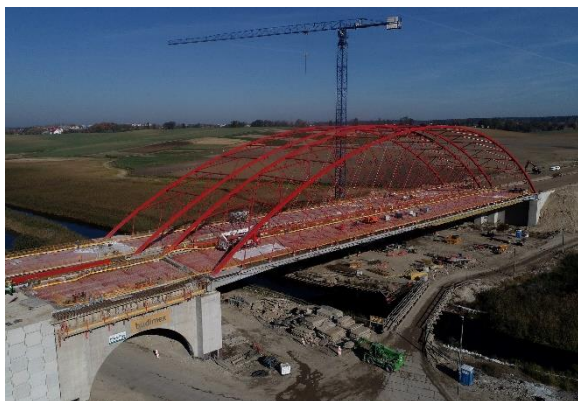
Figure 7. A general view of the bridge - final stage
