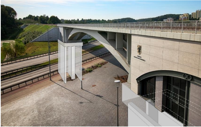
Figure 1. A general view of the railway viaduct WK-11 (photo by Tadeusz Brzozowski)
