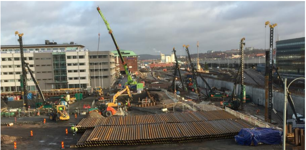
Figure 1 Comprehensive piling is taking place in central Gothenburg
