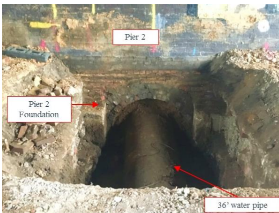
Figure 4. Frontal view of pier 2 with raw water pipe going underneath the arching foundation.
